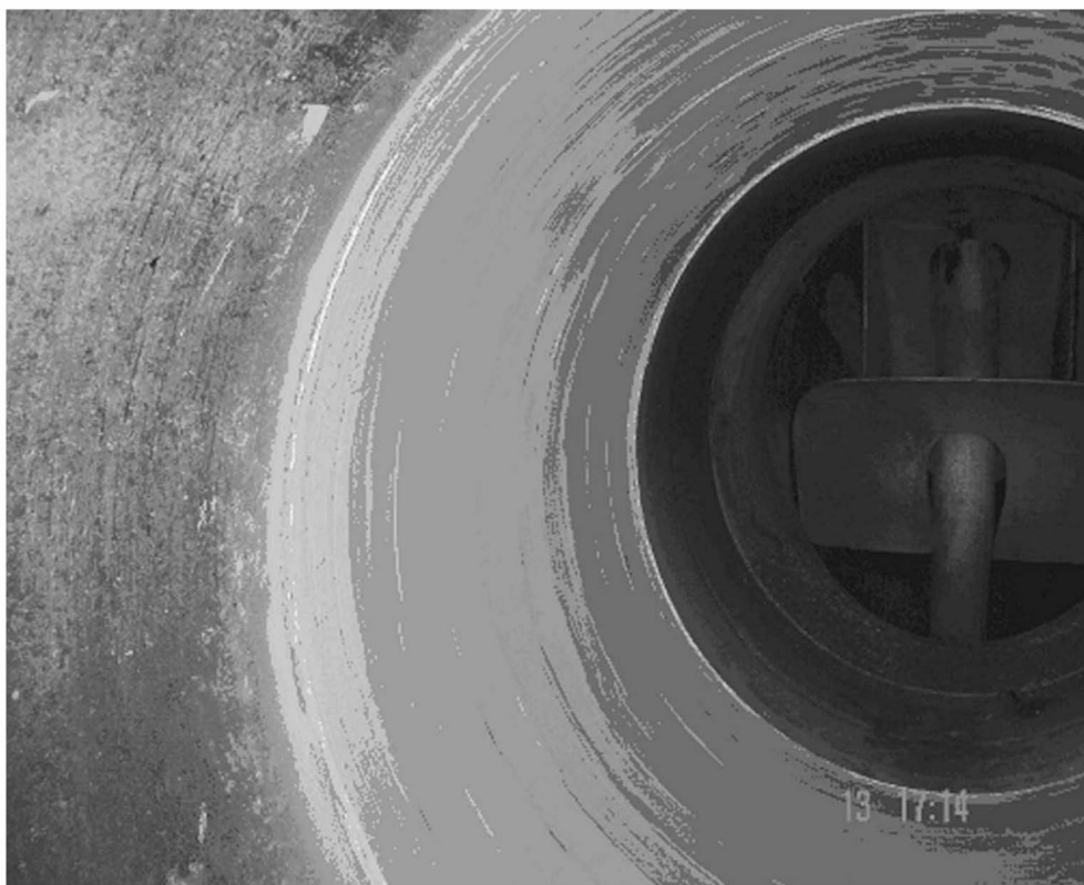
Figure 403-1.1-1 Structural Liner in Raw Water System
