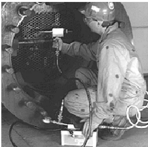
Figure 312-4.2-3 Typical Installation of Mechanical Fit Tube Plugs
